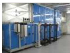
Air Handling Unit ( AHU )
